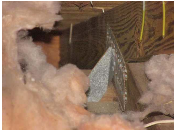
Clips with a minimum of 3 nails
