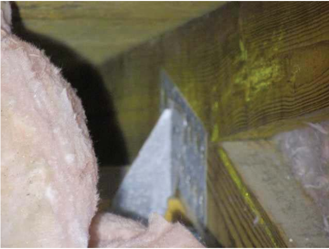
Clips with a minimum of 3 nails
