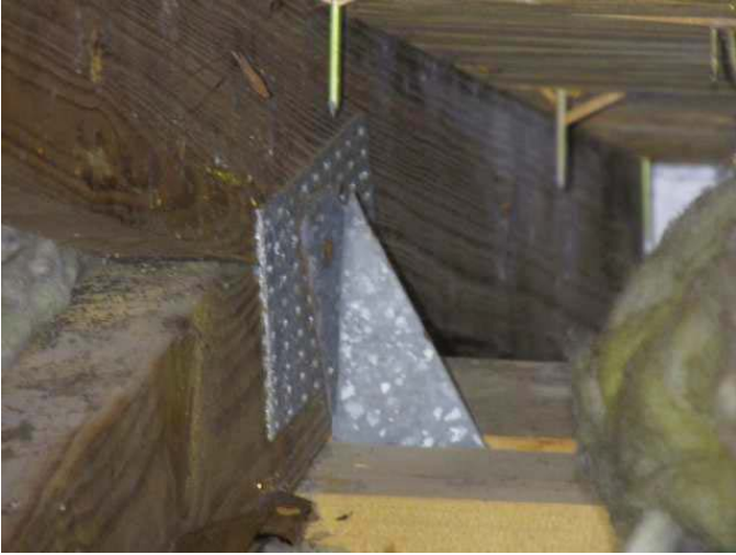
Clips with a minimum of 3 nails
