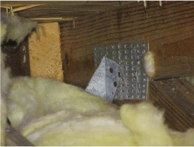
Clips with a minimum of 3 nails
