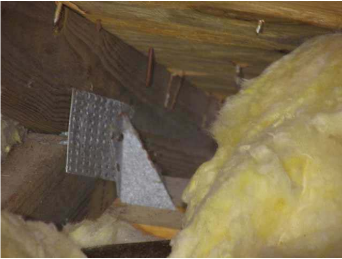
Clips with a minimum of 3 nails
