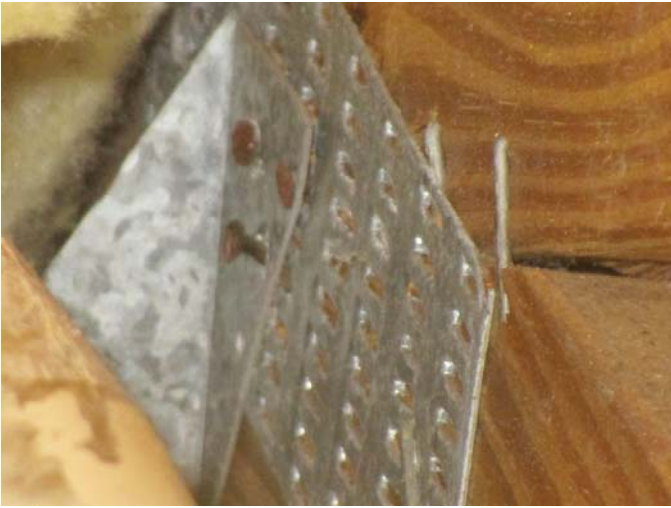
Clips - with minimum three nails
