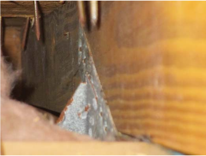
Clips - with minimum three nails
