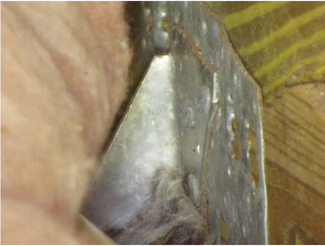
Clips - with minimum three nails
