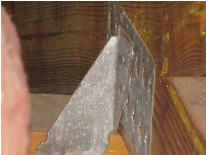
Clips with a minimum of 3 nails
