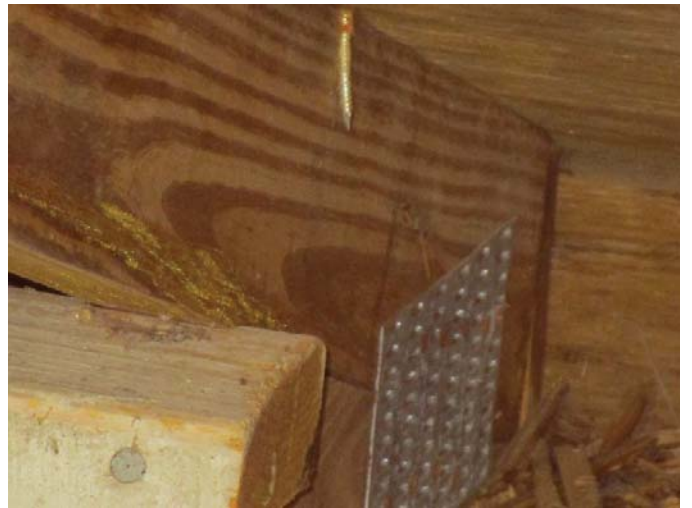
Toe nails - straps do not wrap over only two nails
