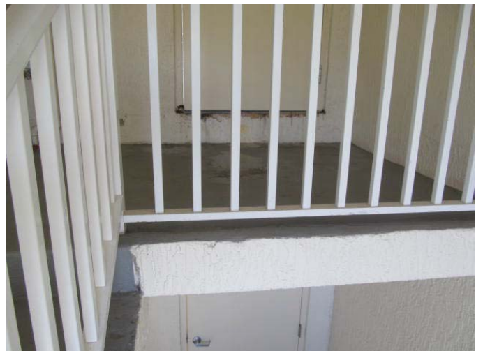
Concrete roof decking
