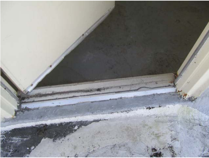
Concrete roof decking
