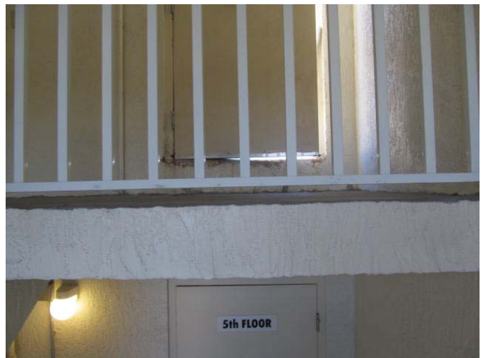
Concrete roof decking
