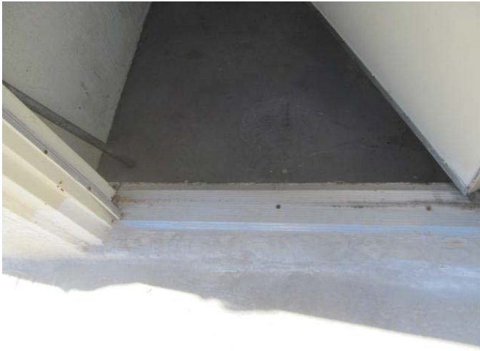
Concrete roof decking
