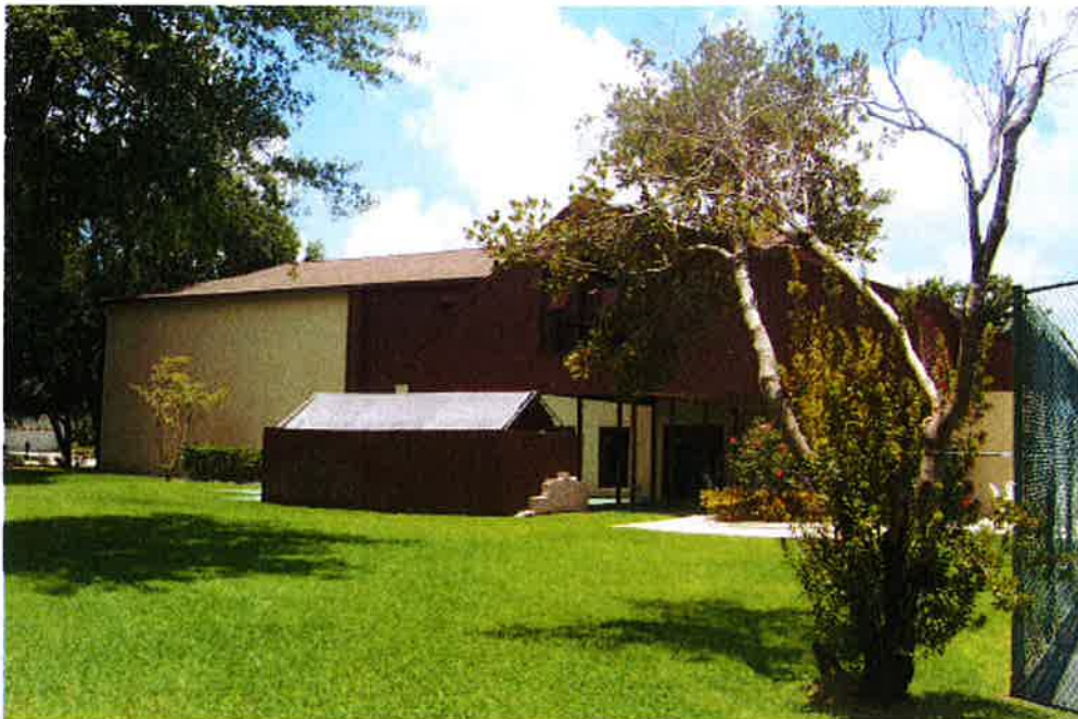
REAR VIEW OF CLUBHOUSE
