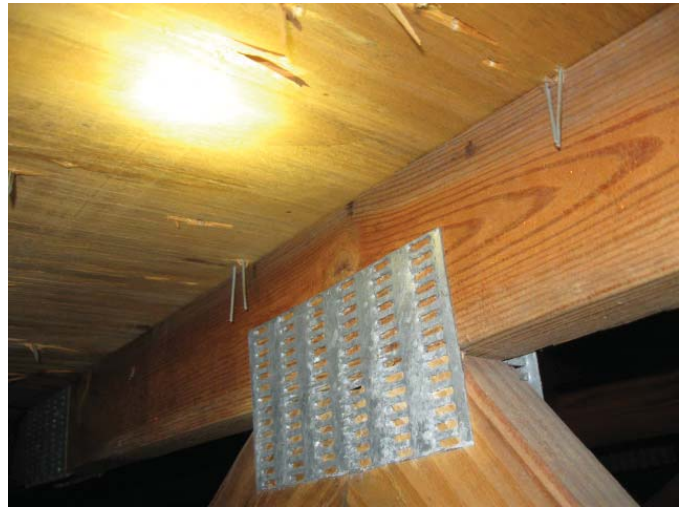
Staples - No evidence of re-nailing found
