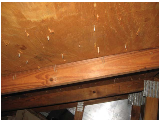
Staples - No Evidence of renailling found
