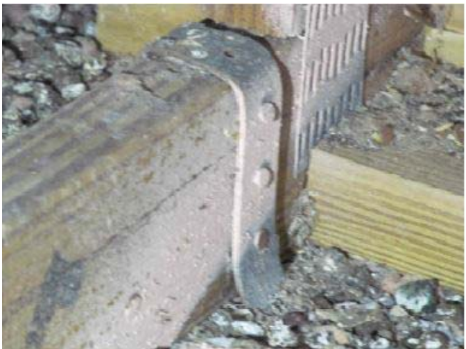
Single wraps - with minimum two nails on front side
