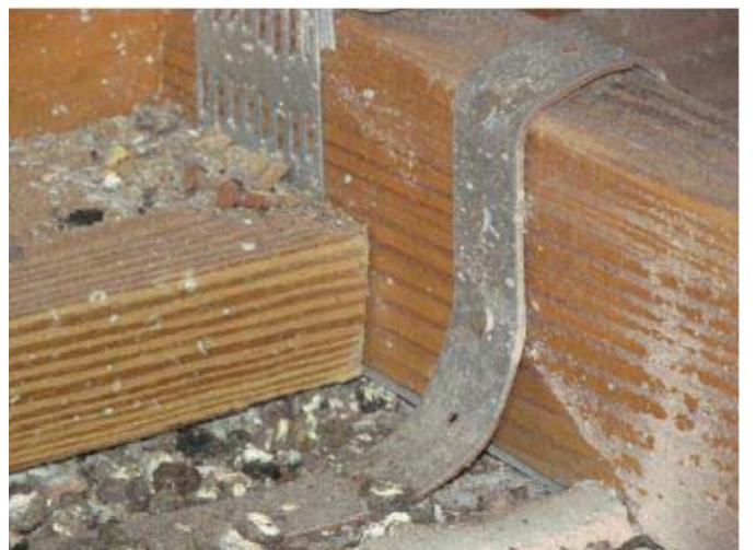
Single wraps - with minimum one nail on opposite side
