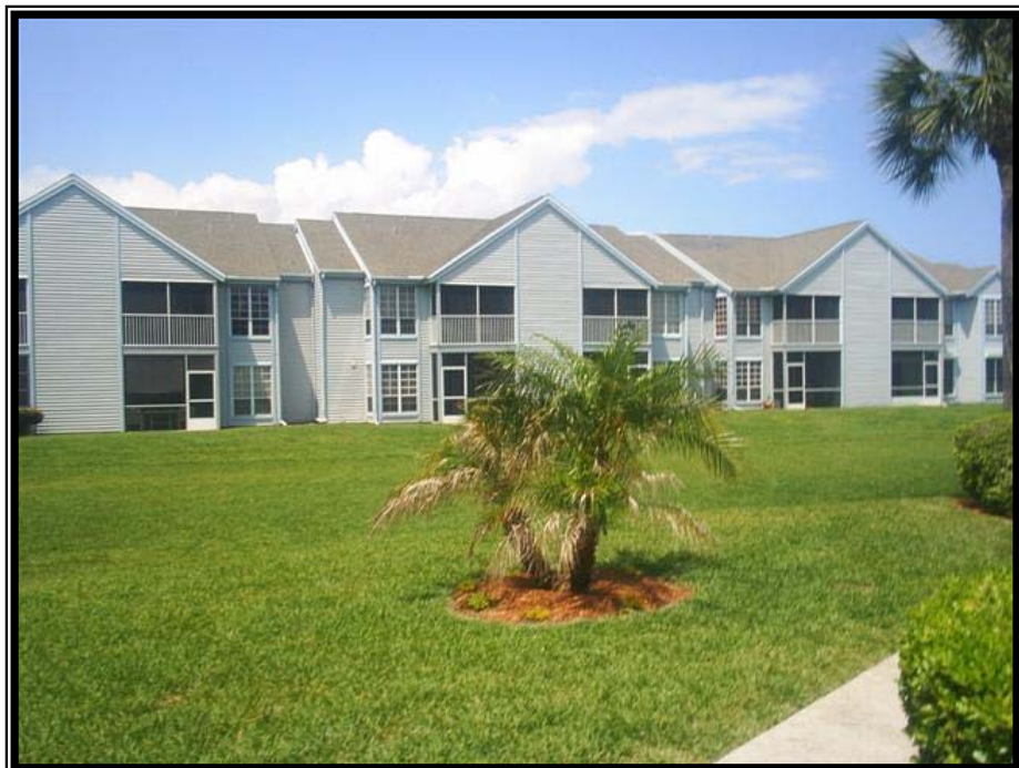
TYPICAL BUILDING - REAR VIEW
