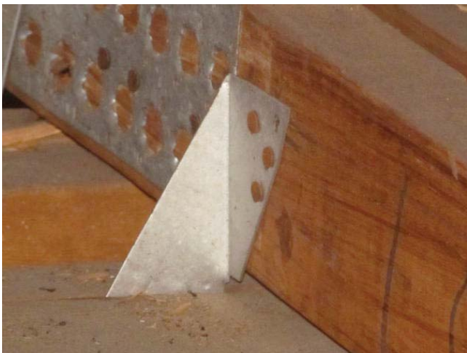
Clips - with minimum three nails
