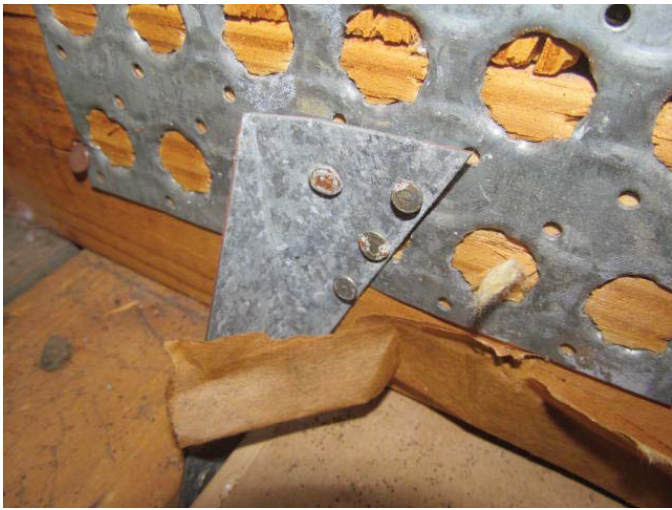
Clips - with minimum three nails
