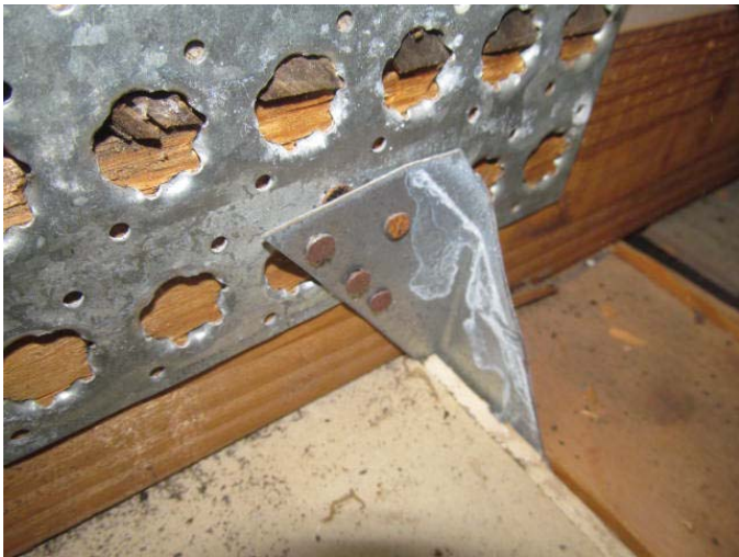
Clips - with minimum three nails
